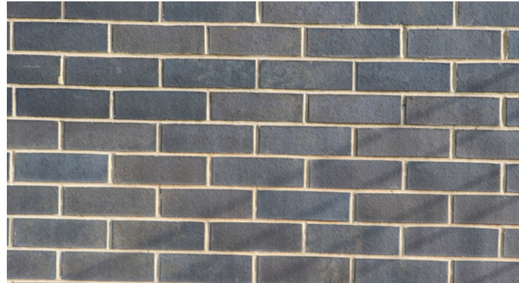
BLUE ENGINEERING BRICKS BELOW DPC
